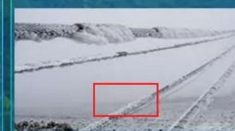
Missing stockbridge damper
