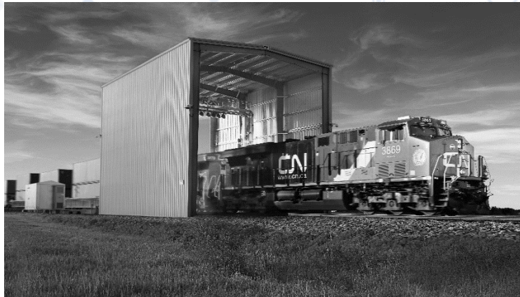
Automated Inspection Portals (AIP)
